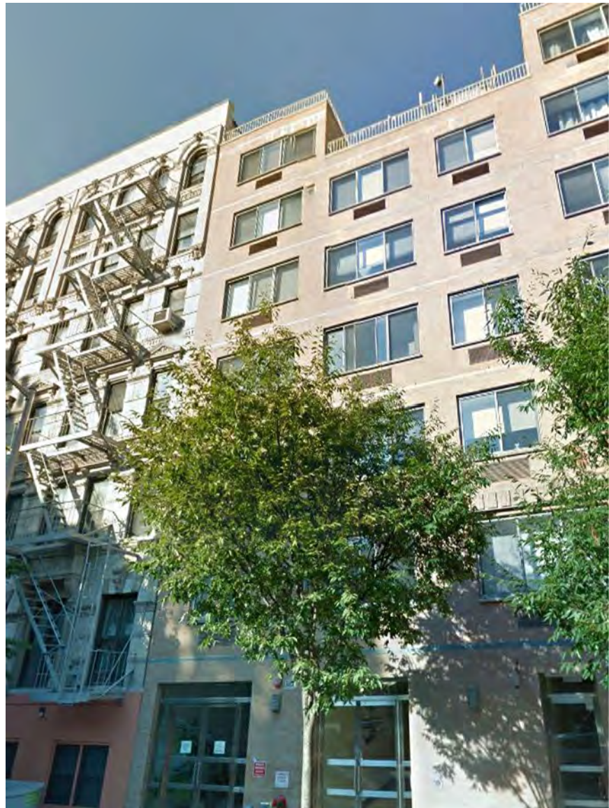
9. VIEW NORTH OF BUILDINGS WEST OF DEVELOPMENT SITE
