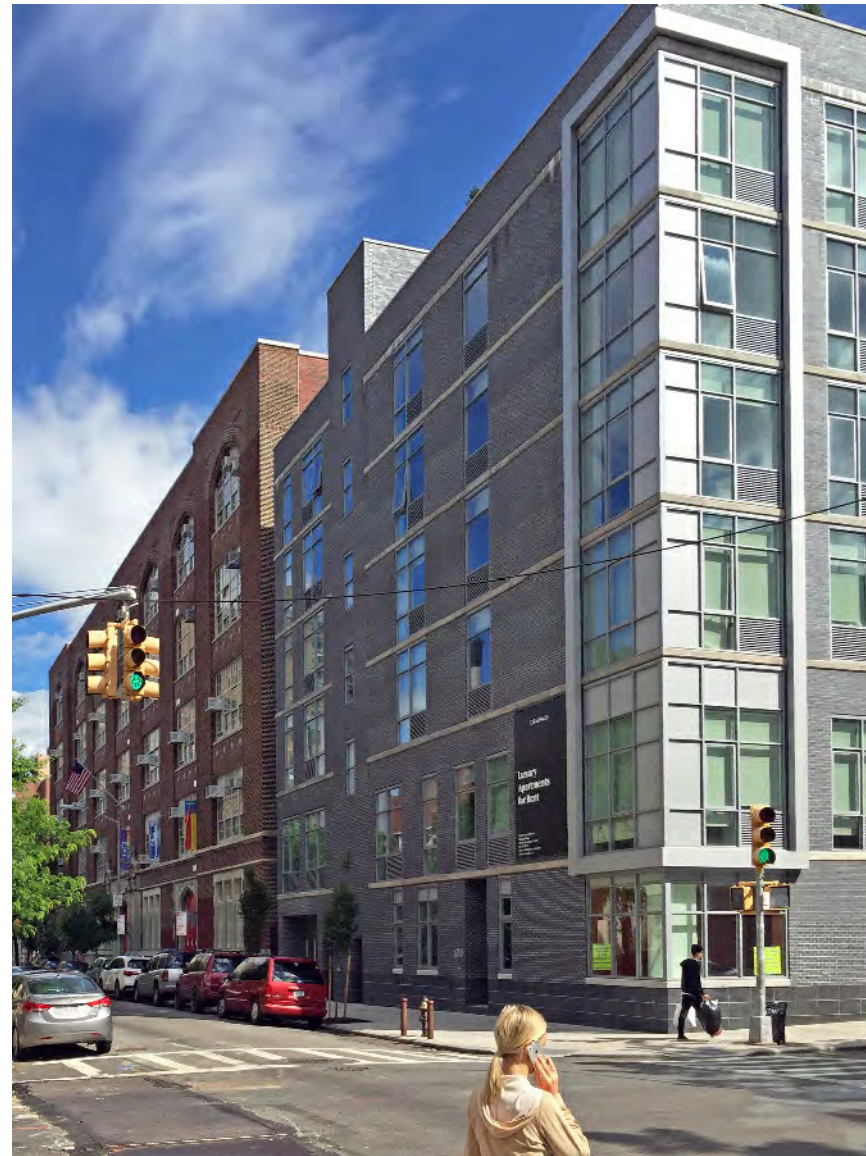
5. VIEW SOUTH EAST OF SOUTHEAST INTERSECTION OF DEVELOPMENT SITE
