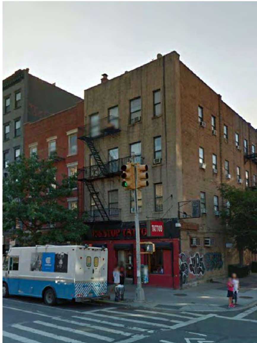
6. VIEW WEST OF THE NORTH INTERSECTION OF THE PROJECT AREA
