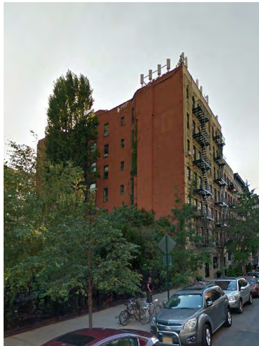
2. VIEW SOUTH WEST ACROSS E 12TH STREET FROM DEVELOPMENT SITE
