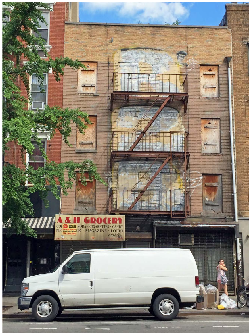
3. VIEW EAST DIRECTLY IN FRONT OF DEVELOPMENT SITE
