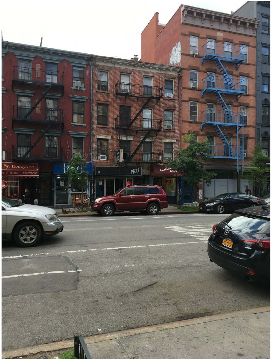
8. VIEW WEST DIRECTLY ACROSS AVENUE A OF THE DEVELOPMENT SITE
