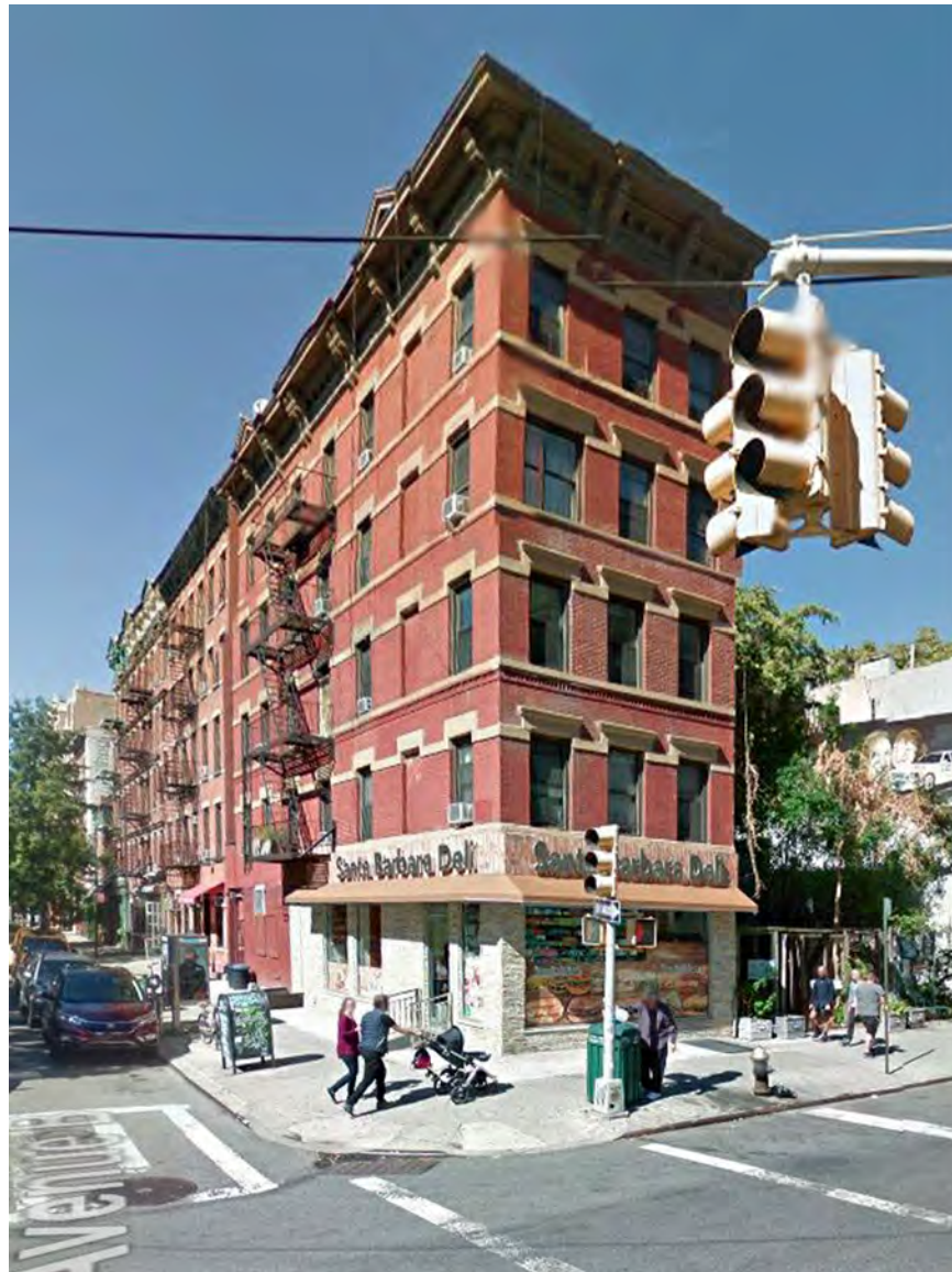
6. VIEW NORTH WEST OF SOUTHEAST INTERSECTION OF DEVELOPMENT SITE
